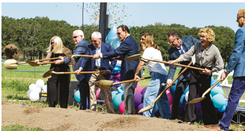
VICTORY Studios: conceptual image (top) groundbreaking (bottom)
